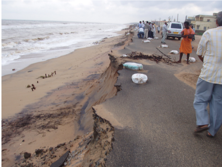
Figure 1 Erosion at Puri in between the Lighthouse & Sterling Hotel beaches (Odisha, India)
