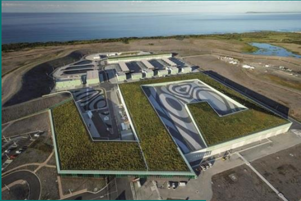
Wonthaggi Desalination Plant, Victoria
